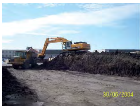
Figure 2: Removal of filling layer
