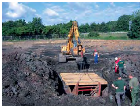
Figure 3: Removal of an unexploded bomb
